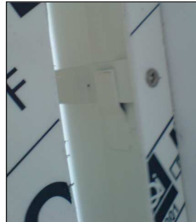
Make sure the brackets slot into the hooks on the mounting frame
