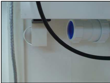
Disconnect flexible hose at the top.
