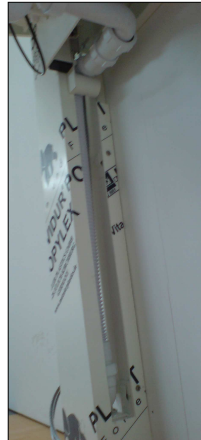
Feed to flexible waste pipe back over the round waste guide brackets and reconnect.
